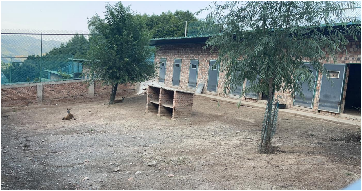
Fig. 1. The overall condition of the enclosure
