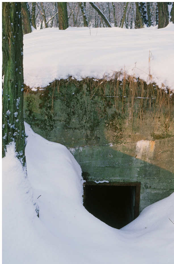
Fig. 1. The entrance to the military shelter under study.
