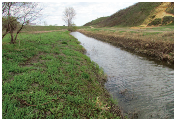
Fig. 6. The drainage canal near Archar, Bulgaria (Fig. 1: 23).
